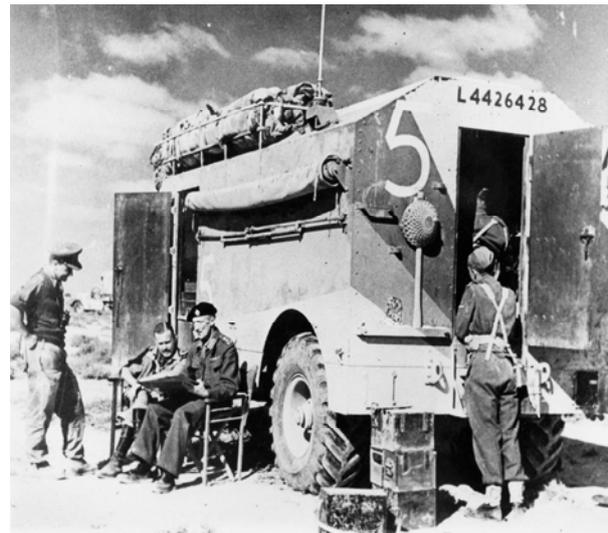
The Associated Equipment Company (AEC) was a familiar truck manufacturer in the UK for many years with its company’s headquarters in Southall, Middlesex. AEC manufactured the Dorchester Armoured Command Vehicle (ACV) that you see in the pictures above. 415 of these vehicles were built. They weighed 12.2 tons and the armour plate was 10-12 mm to provide personal protection from small arms fire. It had a speed of approximately 45 mph.
