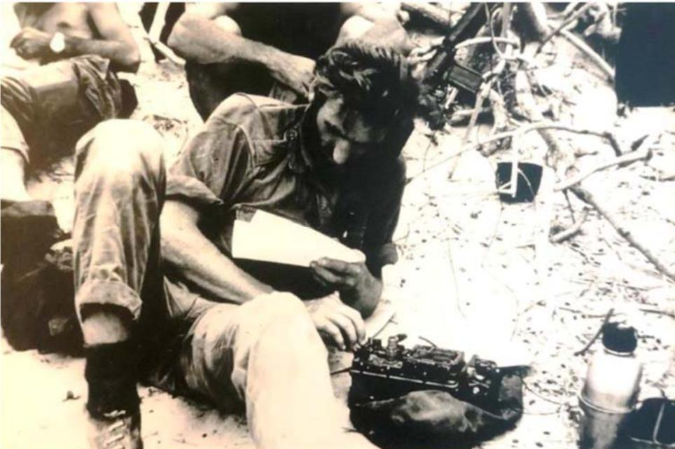
Its low protection from interception meant that later it had to be replaced by more sophisticated sets. However, for its time in operations in Malaya and Borneo it proved to be a very reliable and useful radio. The picture on the left shows it in use on a long distance patrol. This operator did not require the Morse Code Card!
